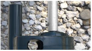
**Step 4:** Now that your greenhouse sidewall EMT conduit is attached to your crank, and the guide EMT conduit is properly installed, you can take your crank and slide it down to where the sidewall EMT conduit meets the guide EMT conduit. From there, simply turn your crank and watch as the crank lifts your greenhouse sidewall!
